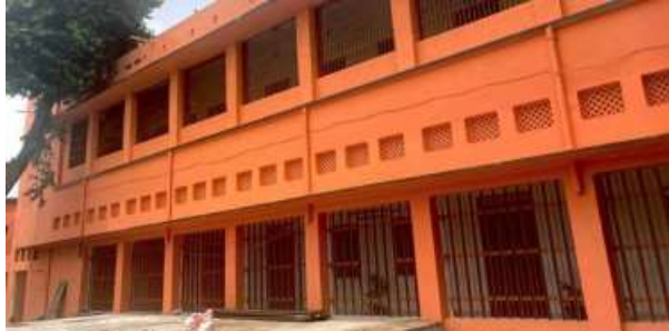
The exterior walls of B.P. Inter School in Begusarai repainted according to the government’s directive. AMARNATH TEWARY
