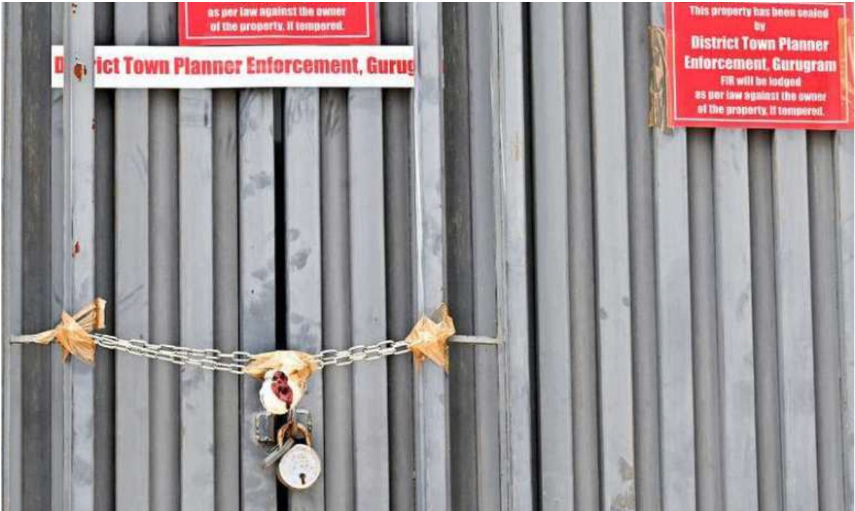
A building sealed by the District Town Planner (Enforcement) in DLF Phase 3, Gurugram on July 6. SHASHI SHEKHAR KASHYAP
