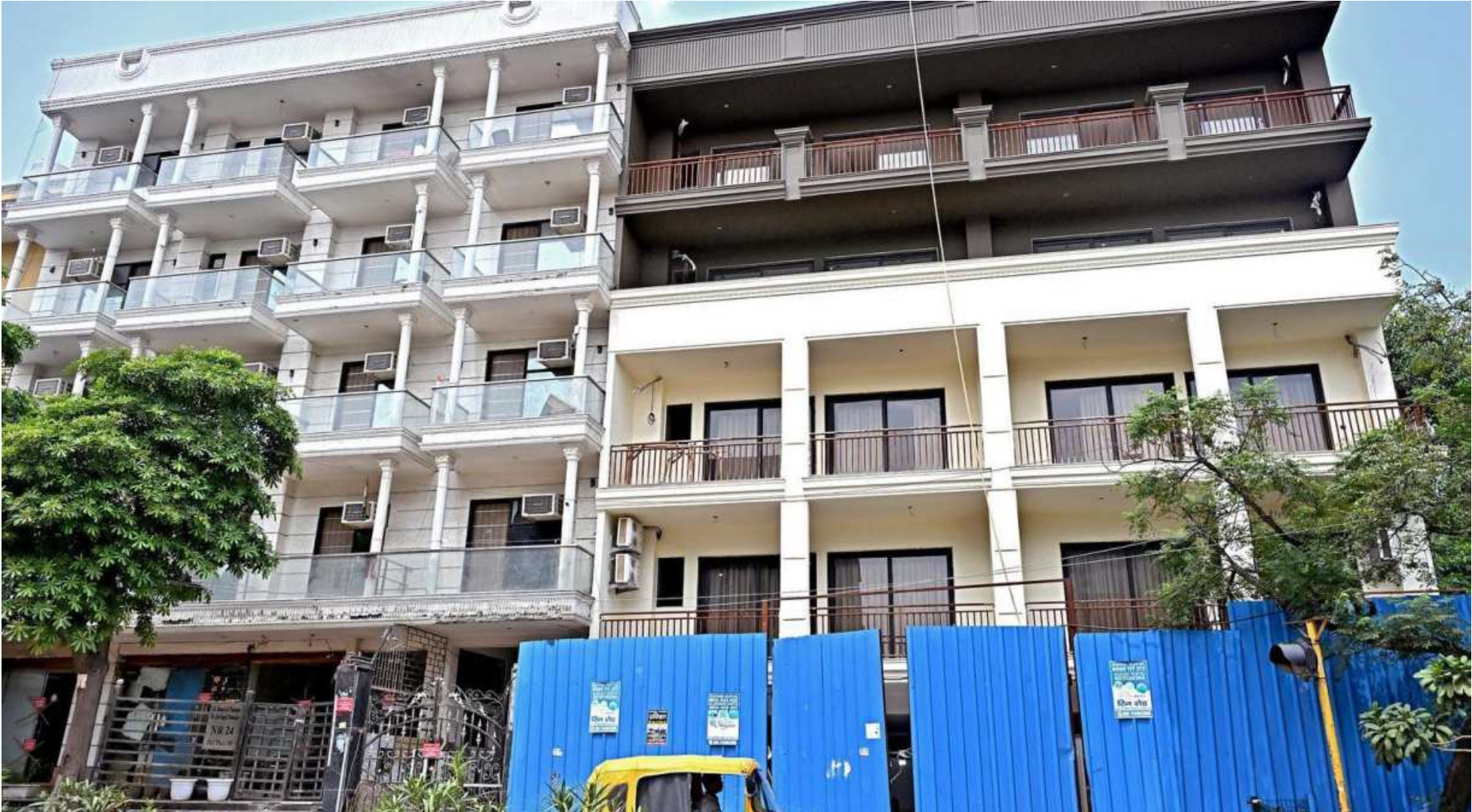
The sealing drive in DLF City Phases 1 to 5 stems from a long-running legal dispute over alleged building bye-law violations, unauthorised constructions and commercial use of residential properties. SHASHI SHEKHAR KASHYAP
