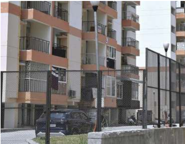
Iron fences at Golf View Condos, Dwarka, Delhi. SHIV KUMAR PUSHPAKAR
