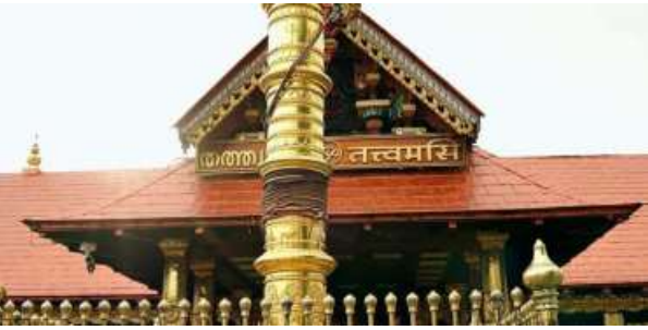
Probe on: The SIT is probing whether fake defects were cited to send the panels at the Ayyappa temple for replating. LEJU KAMAL
