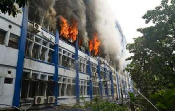
A fire breaks out at a government building in Kolkata’s Alipore area that houses the South 24 Parganas Zila Parishad office. ANI
