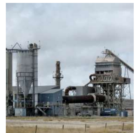
A rotary kiln is visible as the rust-coloured horizontal tube at the centre in this image of a cement plant in the U.S. GREG GOEBEL (CC BY-SA)
